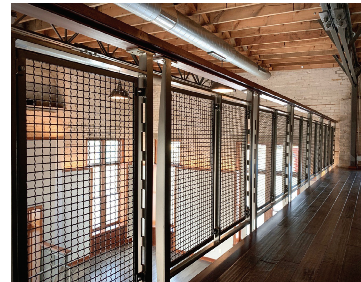
[Bottom Left] The interior structure being stabilized with a temporary steel armature prior to construction. [Top Left] An existing interior condition with punched openings between the two buildings. [Top Right] New bank entrance with reclaimed wood trims and decorative metalwork. [Bottom Right] A new mezzanine framed in the bank with custom steel guardrail.
