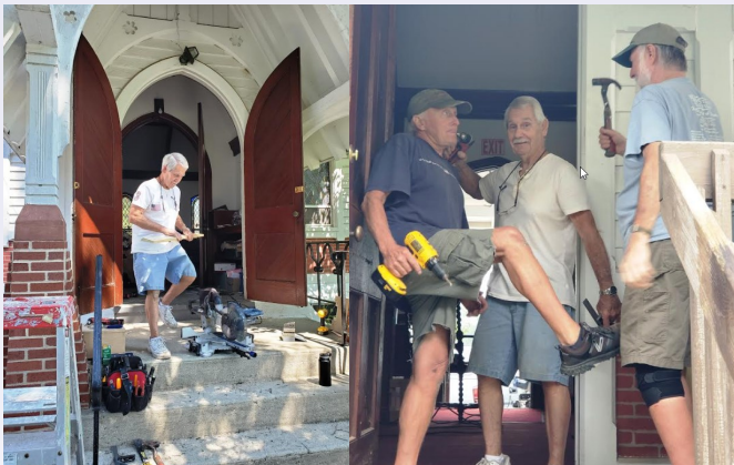
Above: Master Carpenters Roland, Hal, & Jack from the firm of Howard, Fine, & Howard Contractors work diligently to modify the doors to increase the legal capacity of the Church.
