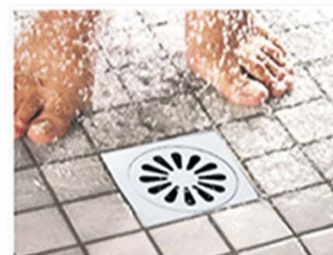
Bathroom floor drain clogged
