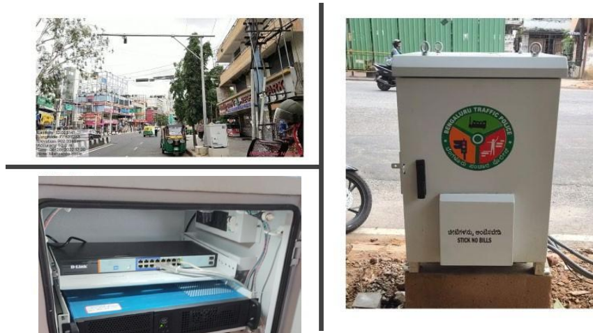
Picture 1. ANPR Camera, Local Processing Unit at an Intersection
