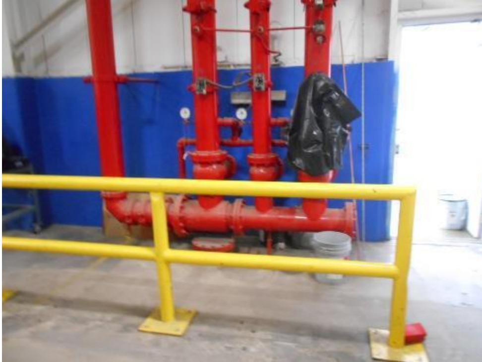
Fire sprinkler risers in Tec Air
