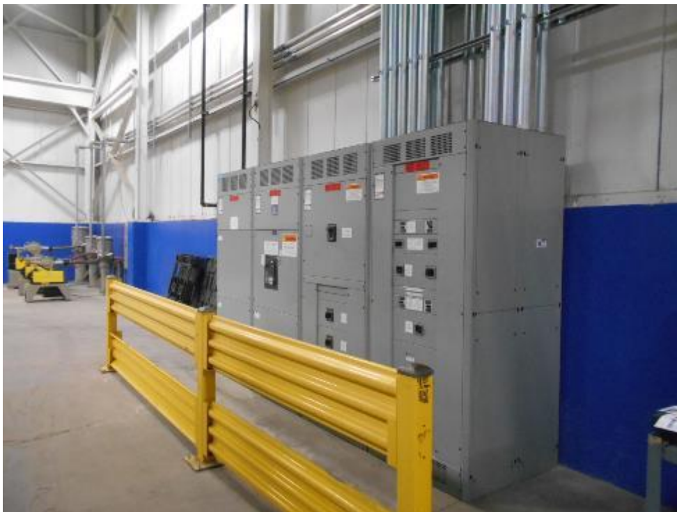
Main electrical service switchgear in Tec Air Premises
