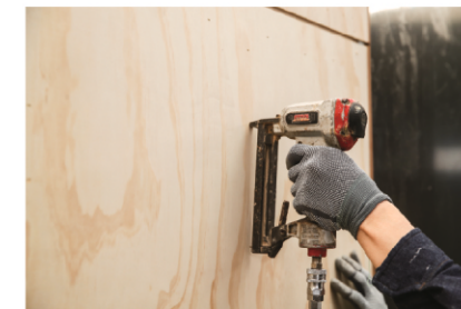
① Prepare the wall Flatness by gypsum board/plywood.
