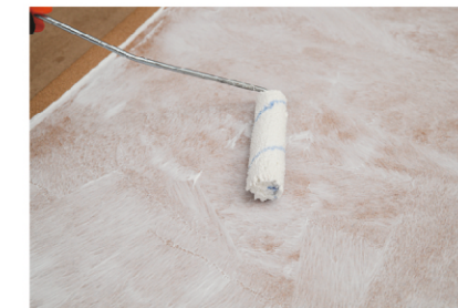
② Spread the Adhesive on a flat surface with a spatula. (Applying silicone to the joints will Enhance the Adhesion.)
