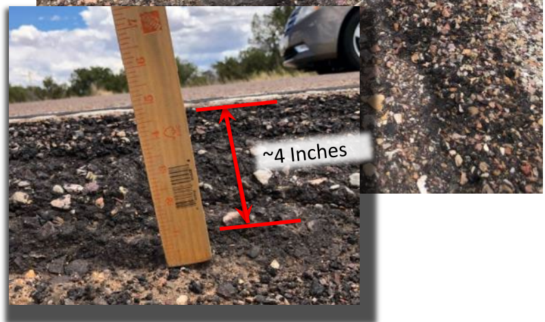
Figure 14 – Pavement Edge Issues
