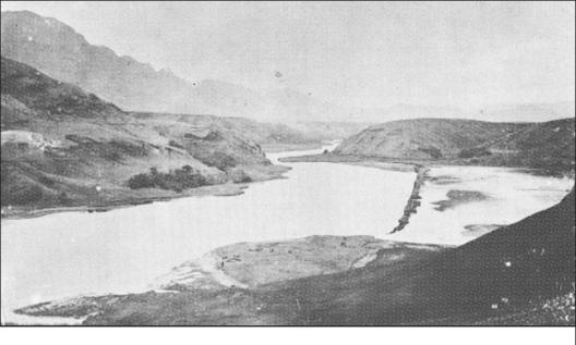
Above photo: An 1890 photo attributed to Theodore P. Severin shows the wall in disrepair with its eastern end broken open.
