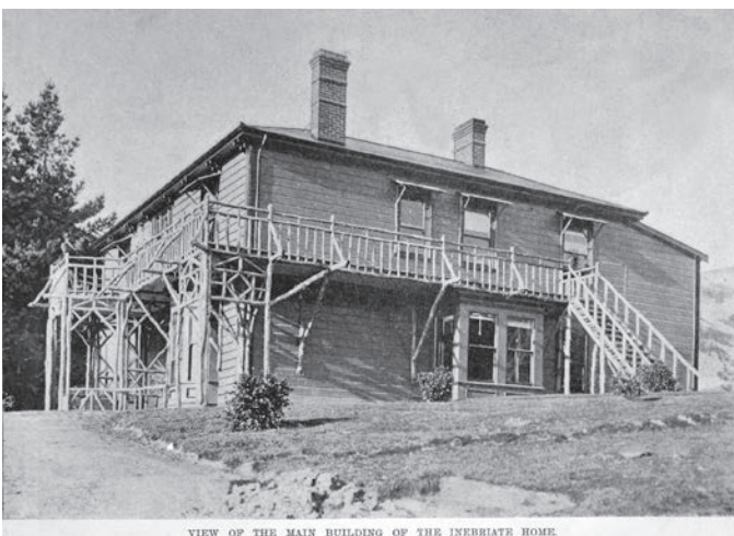
VIEW OF THE MAIN BUILDING OF THE INEBRIATE HOME.
