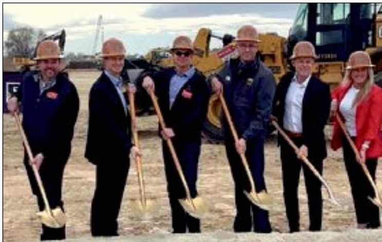
Ground-breaking ceremony including Fred Meyer President Todd Kammerer (left of man with sunglasses) flanked by Mayor Eric Phillips, ESI Construction Management, Corey Barton from Corey Barton Homes, and Kroger Real Estate and Kroger Construction.
