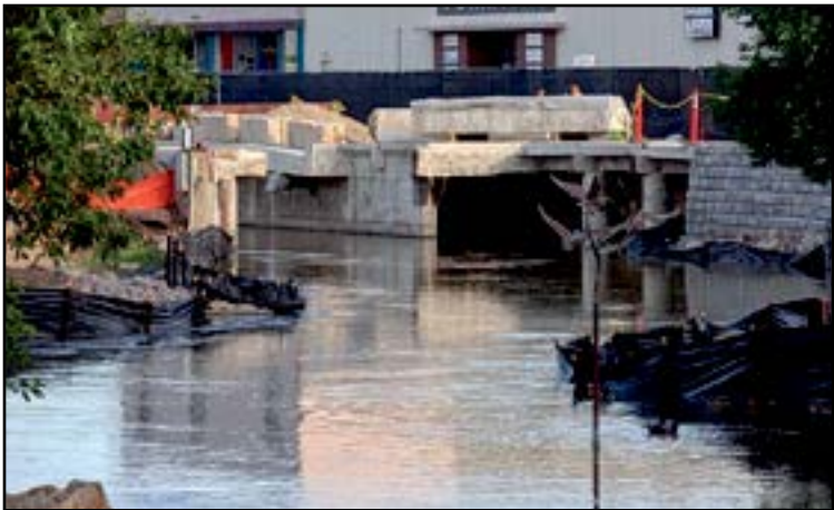
Contractor LaRiviere installed a turbidity curtain along Indian Creek to keep Kimball Bridge construction activities from disturbing the creek. Newly arrived equipment will place large rocks in the creek.
