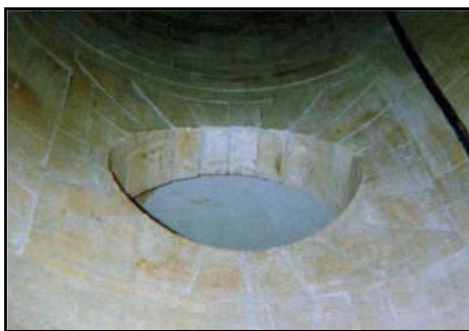
Figure 5. Cylindrical transitions are designed for high temperature lining alignment.
