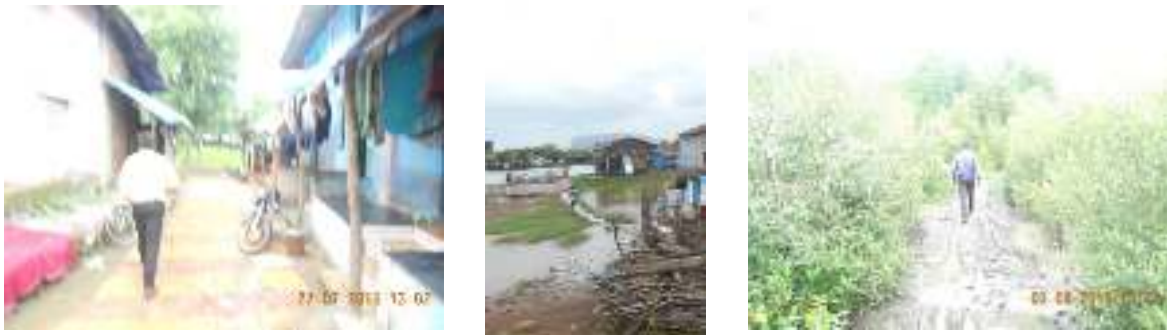
Figure 2-16: Existing Condition of village roads in the interiors
