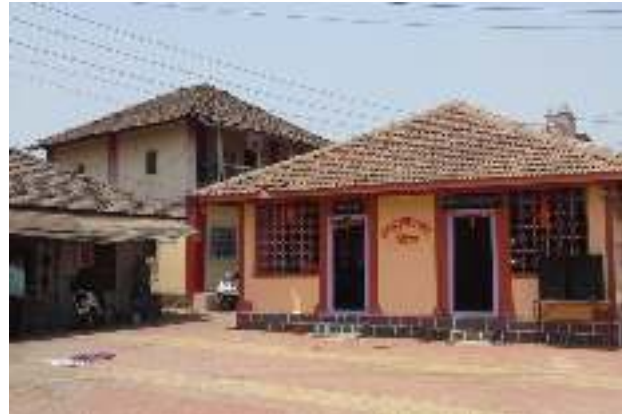
Community Recreational space in front of temple in Vihighar village
