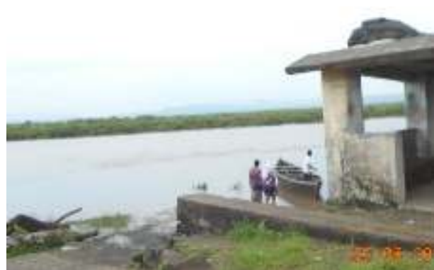
Jetty in Pen Taluka
