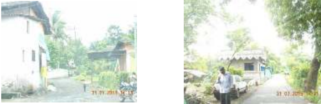
Figure 2-15: Existing Condition of village roads in NAINA
