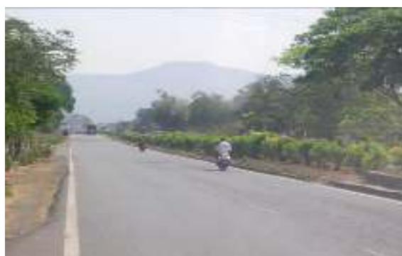
Existing Condition of NH - 04
