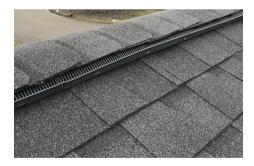
Ridge vent is exactly what it sounds like. The decking at the top of the roof is not installed tightly. There is a gap between each deck, and the ridge is left open. A layer of sponge like material is installed over that gap. Ridge cap shingles are then installed over that venting material. You will notice that the ridge cap is elevated slightly and a gap or black mesh is filling in that gap.
