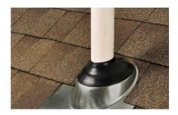
Pipe jacks and split boots are rubber seals that are applied around the roof vent pipes on the roof for the bathroom fans and sewer pipe vents. These are applied over the pipe, and the shingles are woven around them. These prevent water from running down the pipe and entering the dwelling.
