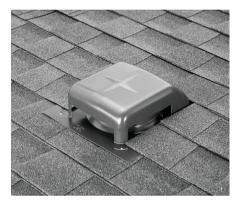
On a roof with vents, holes are cut into the decking, and a vent is applied over the hole. This vent keeps the elements out, but allows air to flow freely in the attic space. The vents installed on these roofs can be either metal or plastic, and they are usually called Turtle vents.
