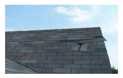
if the wind speeds are very high, it can often tear shingles off the roof, which will leave the underlayment or seal strip of the shingle below it exposed. You can see that here in the photos below. If this happens, it is recommend that a tarp or piece of underlayement be applied over the area to prevent water intrusion.
