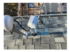
2. Take an overview photo of the accessories, and then a close up of each one. You should try to do this with all accessories, such as vents, skylights, pipe jacks, etc. If the vents are clearly impacted or damaged by hail, you don't have to take a close up of each one, just get an overview and one or two closeups.
