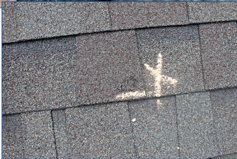
Figure 1 – Example of a hail-caused bruise looking down at the top of an asphalt shingle.
