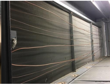
Photo 257 - Averaging Temperature Sensor Element for Supply Air
