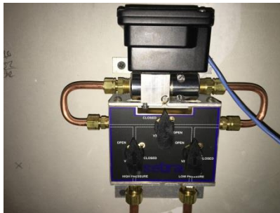
Photo 293 - HDPT with Three-Port Manifold
