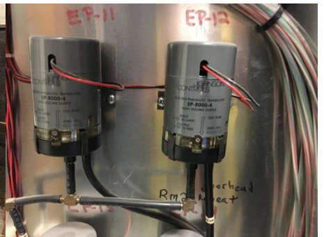
Photo 376 - Johnson Controls Electric to Pneumatic Transducer
