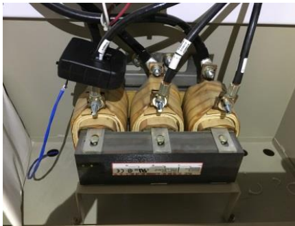
Photo 281 - Current Transmitter Installed on a Water-Cooled Chiller
