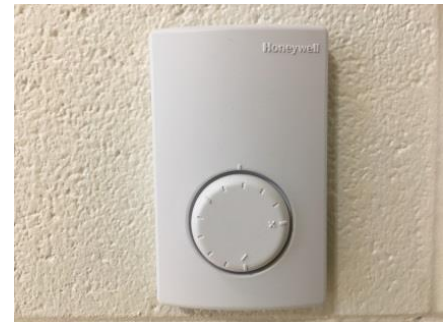
Photo 252 - Space Temperature Sensor with Setpoint Adjustment
