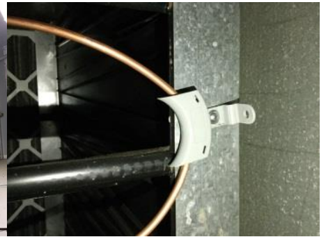
Photo 258 - Averaging Temperature Sensor Support
