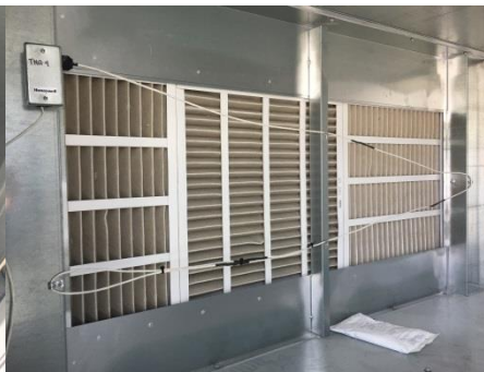
Photo 260 - Flexible Averaging Temperature Sensor at Filter
