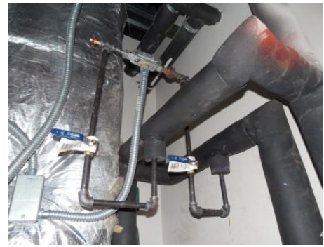
Photo 297 - Thermal Trap Installed to Prevent Condensation
