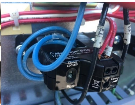
Photo 206 - Additional Loops Around CSR Core
