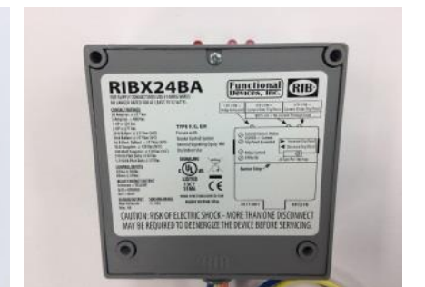
Photo 210 - RIB® Relay With Internal Current Sensing Relay
