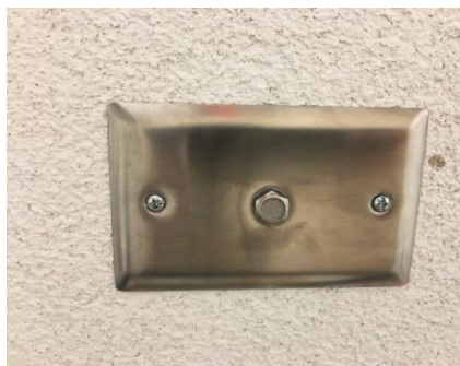
Photo 290 - Ceiling or Wall-Mount Space Static Pressure Pickup
