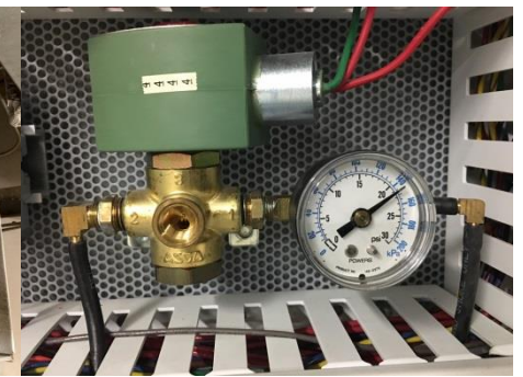
Photo 355 - 24 VAC Solenoid Air Valve
