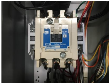
Photo 66 - Magnetic Contactor
