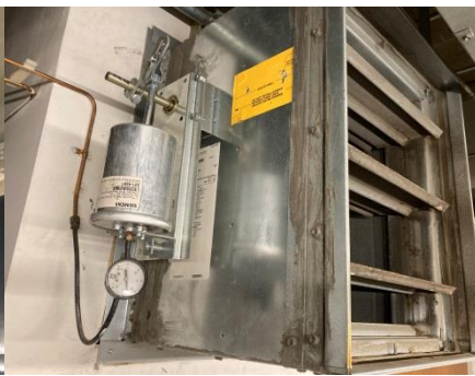
Photo 354 - Pneumatic Two-Position Outdoor Air Damper Actuator
