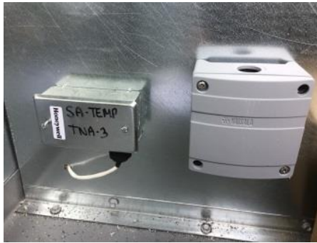
Photo 256 - Flexible Averaging Temperature Sensor (Left)
