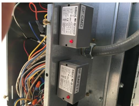
Photo 71 - Enable and Safety Relays Example #1
