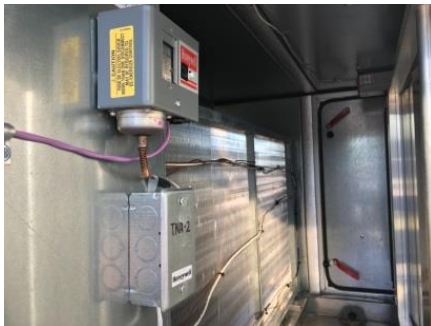
Photo 190 - LTD Installation Inside of AHU
