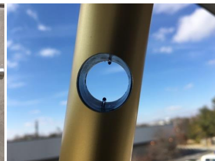
Photo 330 - Close-up View of Photo 331 - Thermal Dispersion Probes
