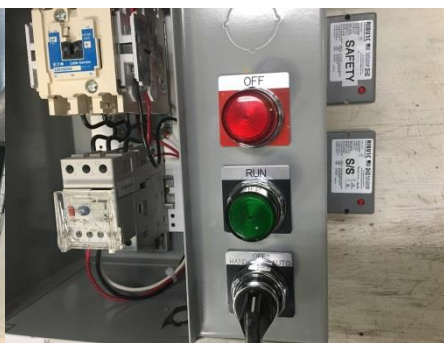
Photo 72 - Enable and Safety Relays Example #2
