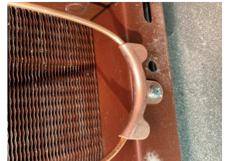
Photo 192 - LTD Mounting Clip Example
