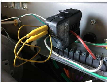
Photo 104 - Magjumper™ on a Current Sensing Relay Contacts
