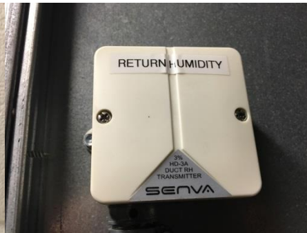
Photo 278 - Duct-Mounted Humidity Transmitter
