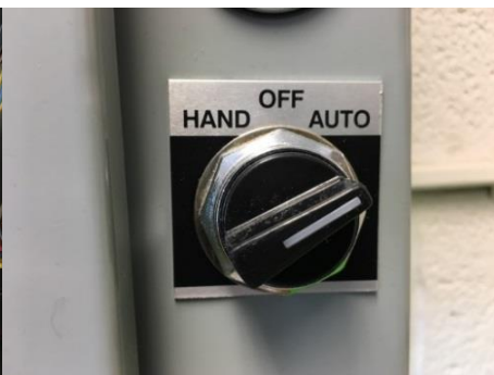
Photo 69 - Hand-Off-Automatic Switch
