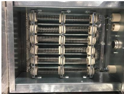
Photo 381 - Slip-in Open-Coil SCR Electric Duct Heater
