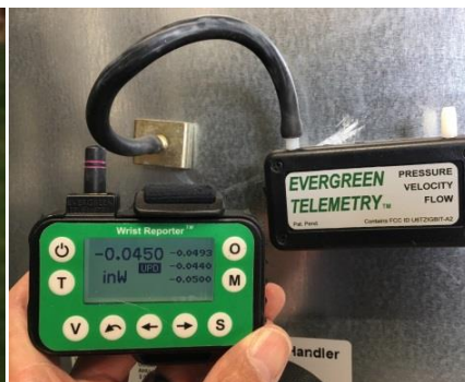
Photo 164 - Pressure Module for Duct Static Pressure Readings
