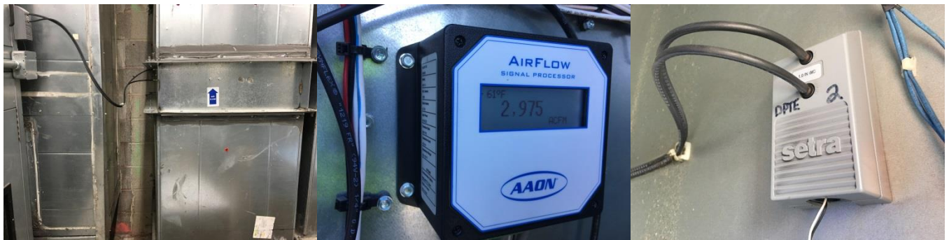
Photo 298 - Duct-Mounted AFMS Installation
