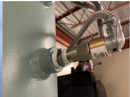
Photo 273 - Immersion Temperature Sensor (Large Diameter)
