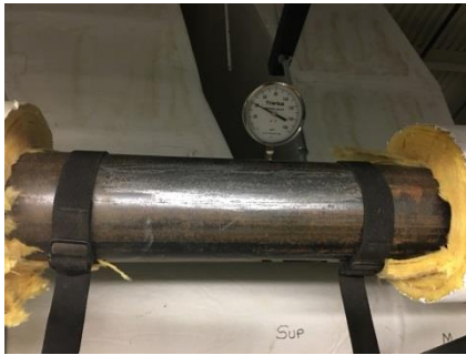
Photo 142 - Insulation Removed and Pipe Surface Prepared
