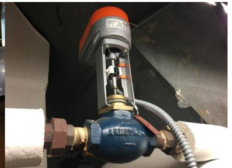
Photo 337 - Steam Globe Valve with Position Feedback
