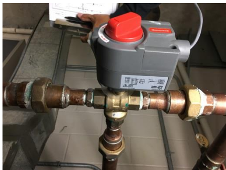
Photo 365 - Modulating Electric Valve Actuator
