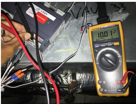
Photo 25 - 100% Valve Command (10.0 VDC Output Signal)
