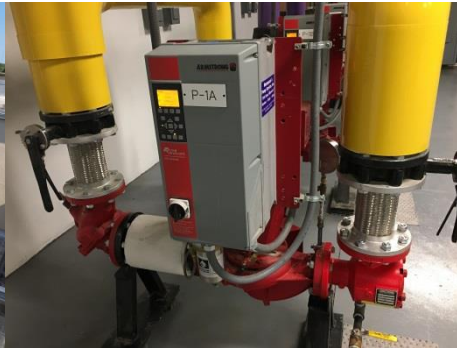
Photo 387 - Dual-Temperature Pump Speed Control
