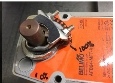
Photo 367 - Modulating Electric Damper Actuator
