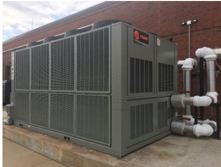
Photo 13 - Air-Cooled Chiller
