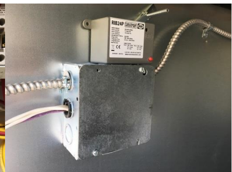
Photo 58 - RIB24P for Electric Resistance Heater Control
