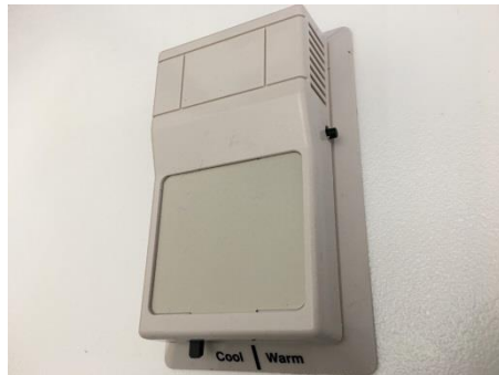
Photo 265 - Space Temp. Sensor with Setpoint Adjustment & Override
