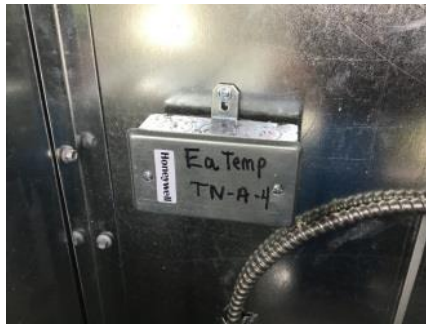
Photo 254 - Probe Temperature Sensor (Monitoring Adjacent Chamber)
