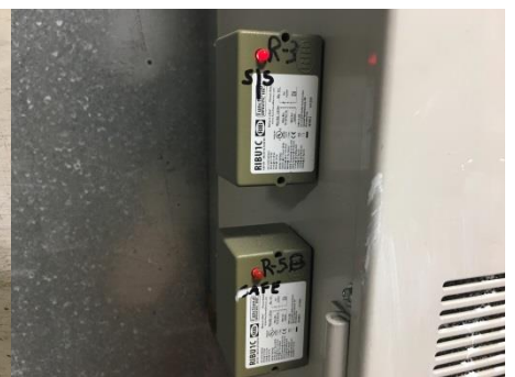
Photo 73 - Enable and Safety Relays Example #3
