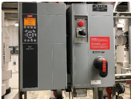
Photo 16 - Variable Frequency Drive
