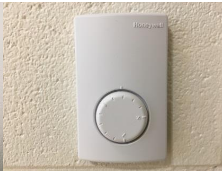
Photo 266 - Space Temperature Sensor with Setpoint Adjustment
