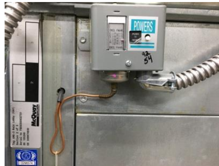
Photo 191 - LTD Installation Outside of AHU
