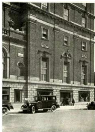
DETAIL OF END BAY
