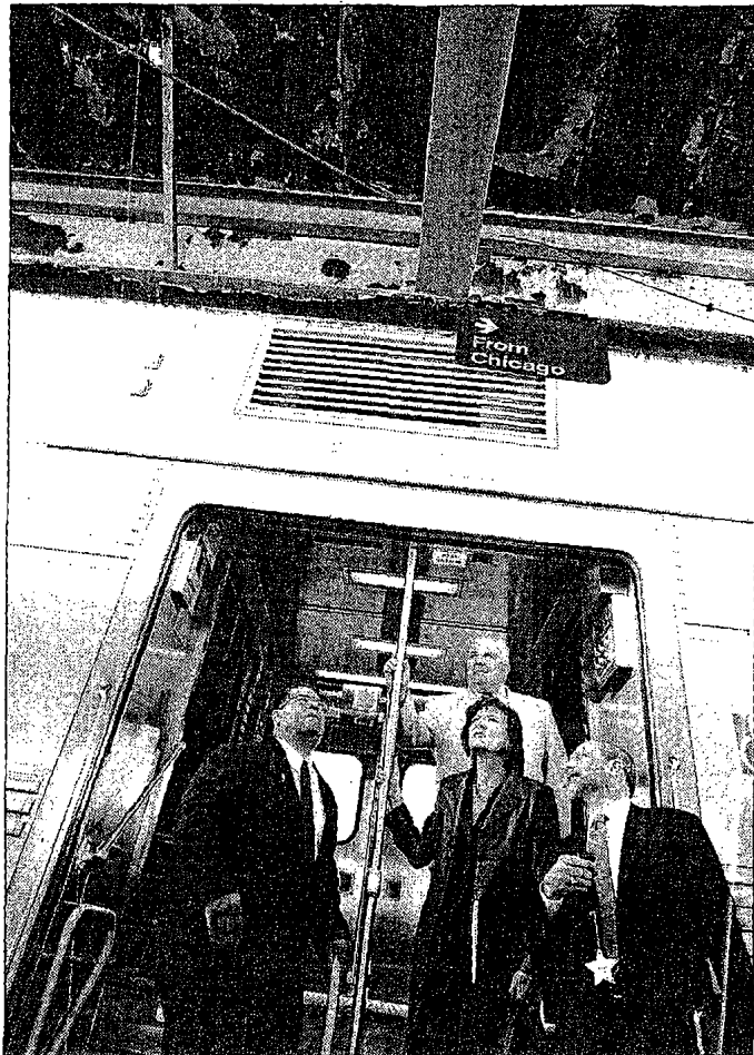
State legislators and transit officials inspect a crumbling roof shelter at the Metra stop in Cicero. ANTONIO PEREZ/TRIBUNE PHOTO
