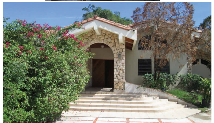
Work begins on the boundary wall and house interior. View of the main house.
