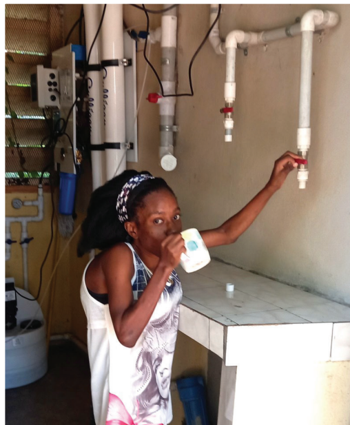
One line from the new water system flows to the showers, kitchen and bathrooms, a second with ultraviolet treatment is used for drinking. Here resident Judith Telus samples the new, fresh water.
