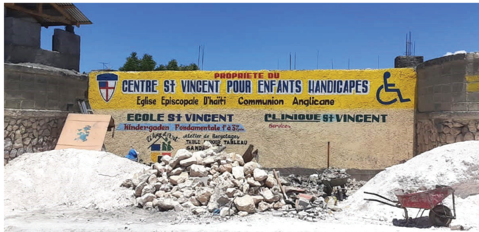
Left: Guard stands on duty in the new security tower at Santo 17. Above: The new replacement wall at Santo 17 makes sure everyone understands who owns the property behind the wall. Gangs broke through this wall and illegally claimed the open land at Santo 17 as their own. Legal action taken by St. Vincent's and support from the police enabled us to secure the property and show force against future incursions.
