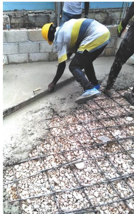
*The workers pour concrete to build the platform for a large, new electrical generator at the Medical Center*
