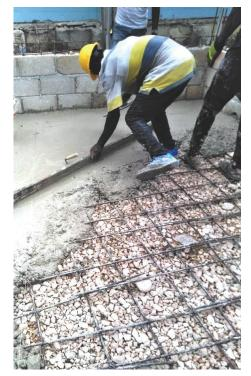
The workers pour concrete to build the platform for a large, new electrical generator at the Medical Center
