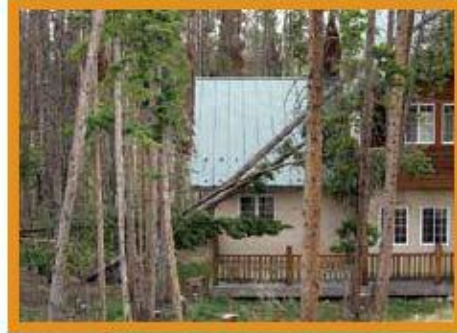
Figure 21: During high winds, these lodgepole pine trees fell onto the house. Lodgepole pine is highly susceptible to windthrow. Photo: CSFS
