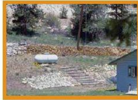
Figure 19: Keep firewood, propane tanks and natural gas meters at least 30 feet away from structures. Photo: CSFS
