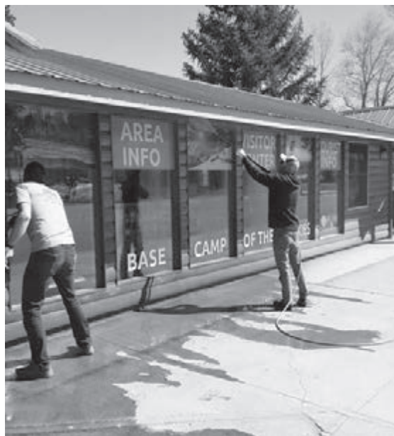
Crews sprucing up the Visitor Center.
