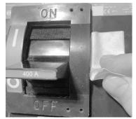
Clean dust and oils from circuit breaker lockout mounting area using an isopropyl alcohol wipe.
