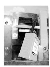
Note: The lockout device is designed to store the locking pins inside the device when not in use. A second locking pin is provided for convenience.
