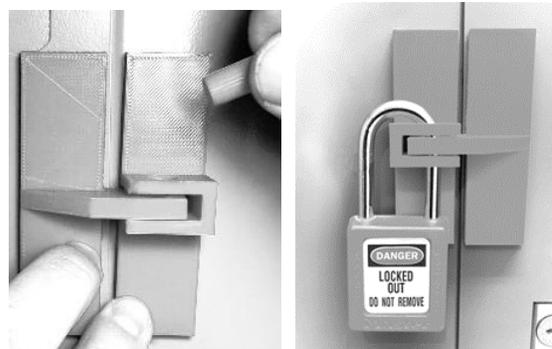
Remove the plastic alignment pin and install a padlock to secure all breaker positions within the electrical panel.
