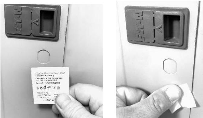
Clean dust and oils from circuit breaker panel cover and door face using an isopropyl alcohol wipe.
