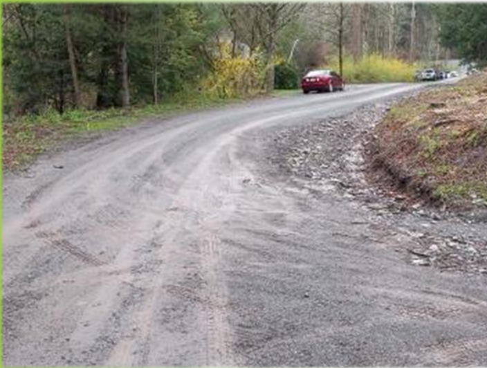
Picture 1: Taking picture near inlet of pipe under road showing where the water leaves the channel & begins flowing down the road.
