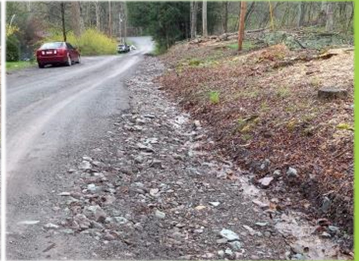
Picture 2: Road Ditch that is badly eroded and showing where houses are along road that get flooded.
