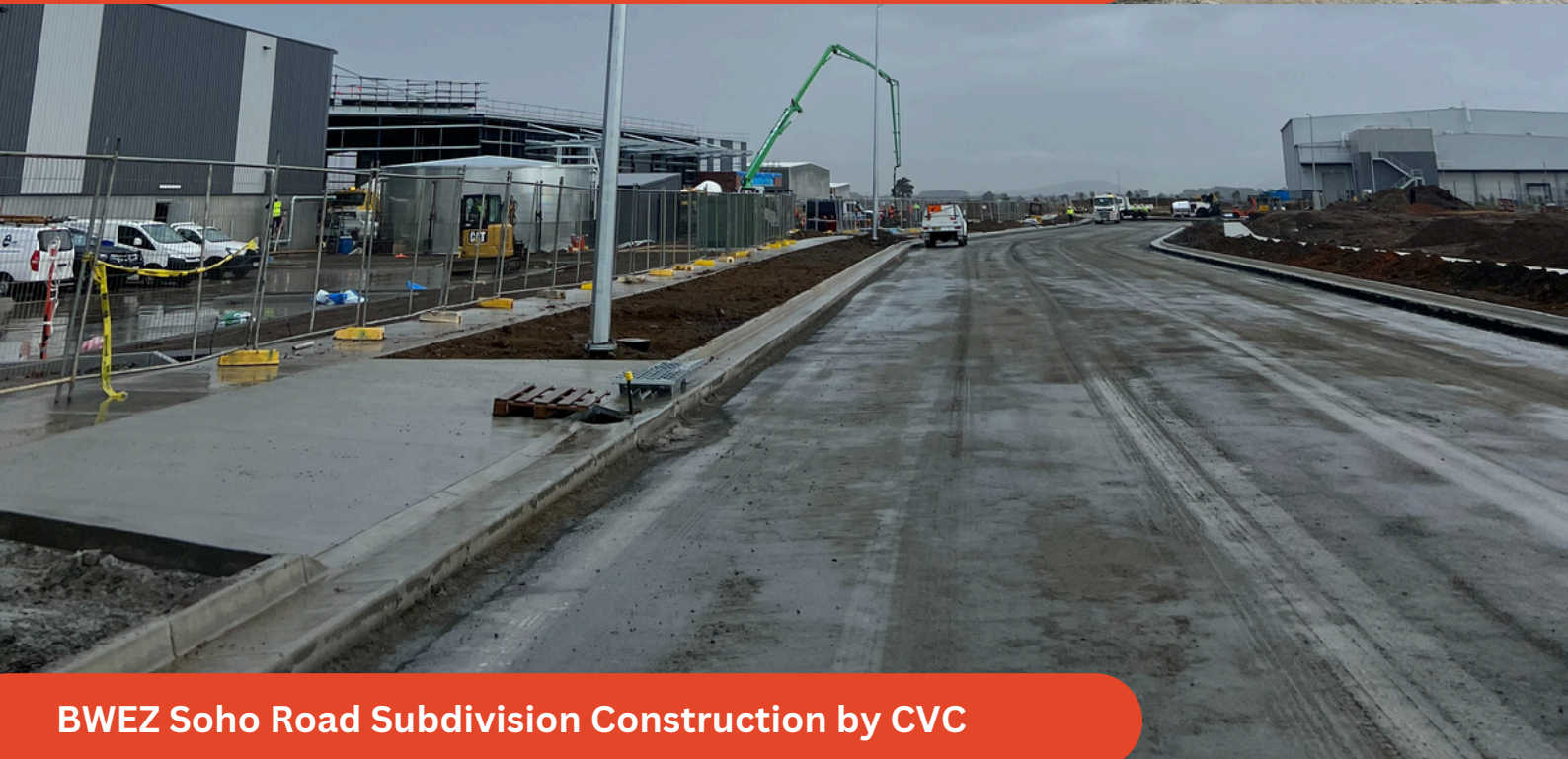
BWEZ Soho Road Subdivision Construction by CVC
