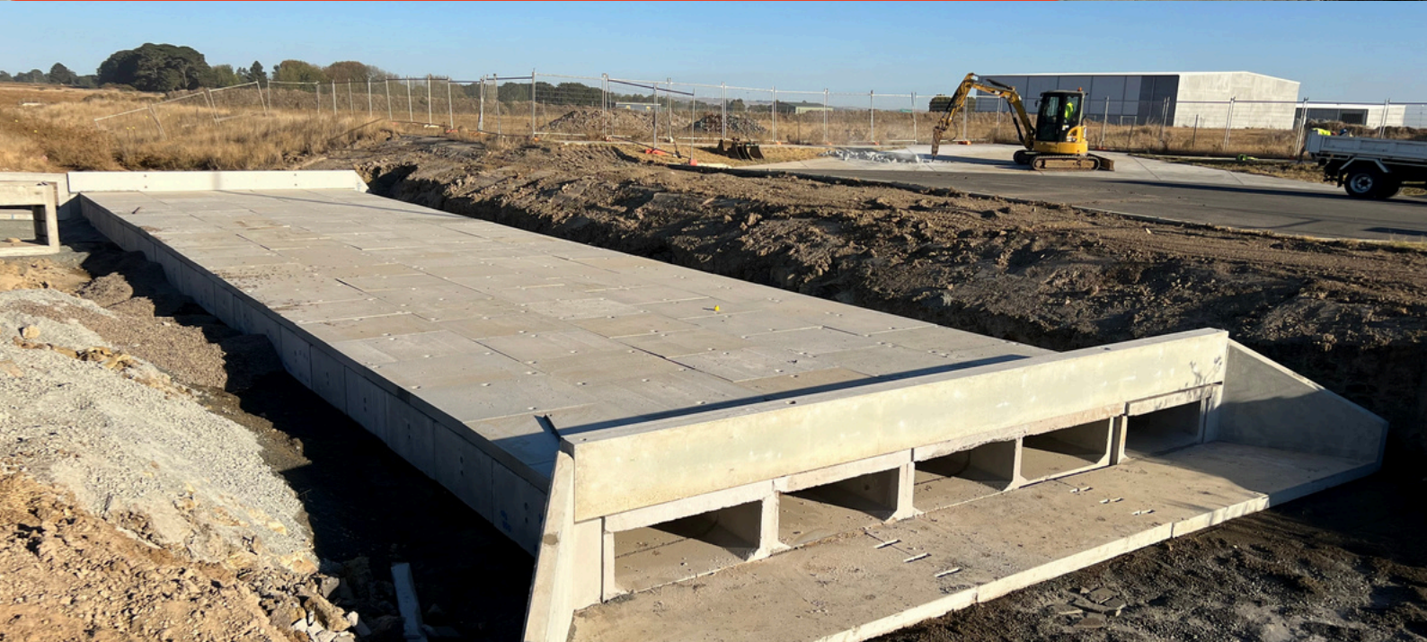
BWEZ Culvert crossing constructed by CVC
