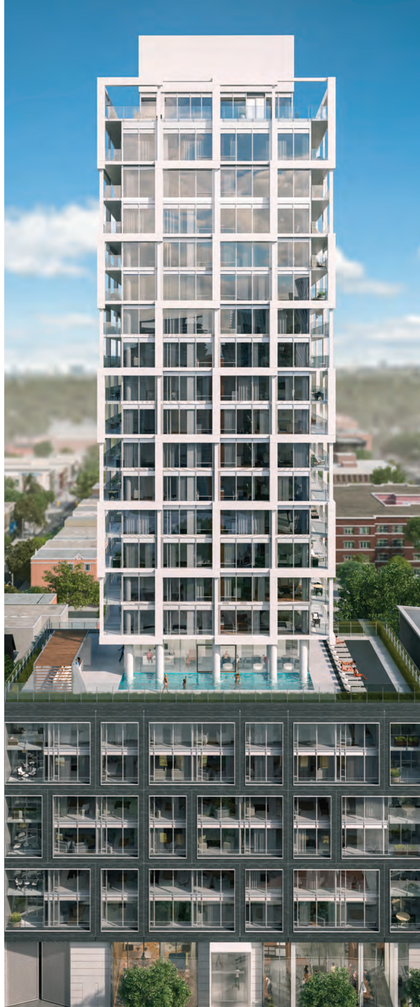
EAST FIFTY FIVE, TORONTO UNDER CONSTRUCTION
