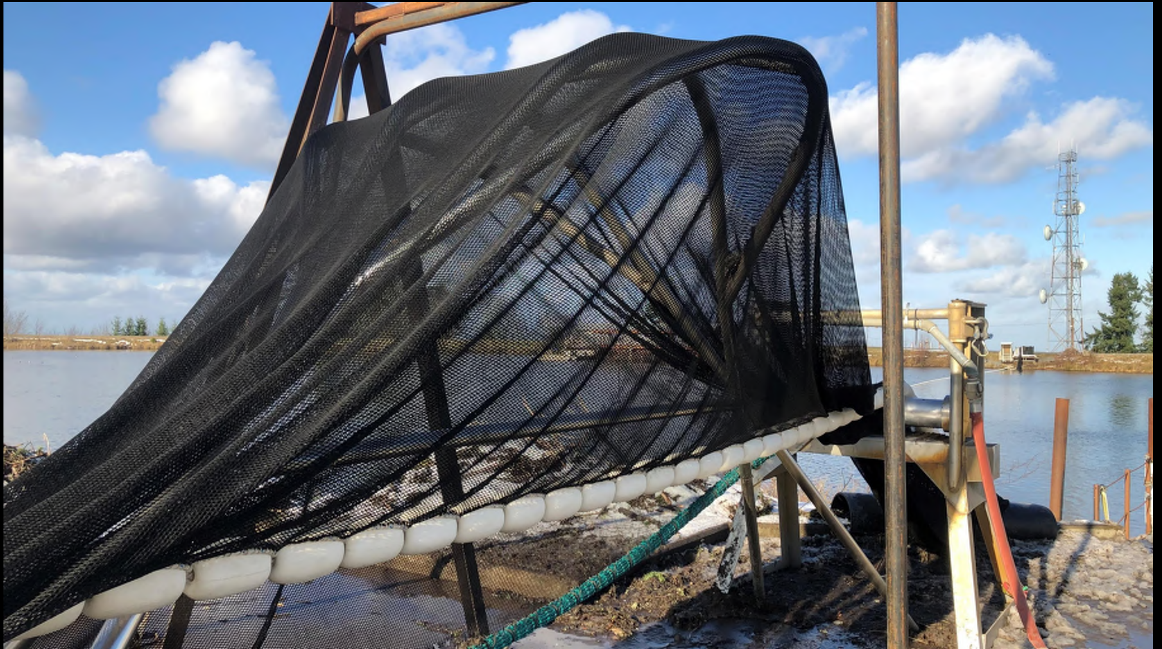
New fish guide/barrier net with increased floats and lead line for efficiency
