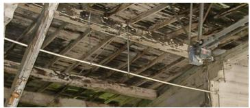
Above: The dark areas of the ceiling in the car restoration area of the roundhouse are not from "old age" but rather the accumulated soot from the steam locomotives serviced here 100 years ago. You can even see the soot from the smokestacks of Rock Island steam locomotives on the ceiling of the conference room!
