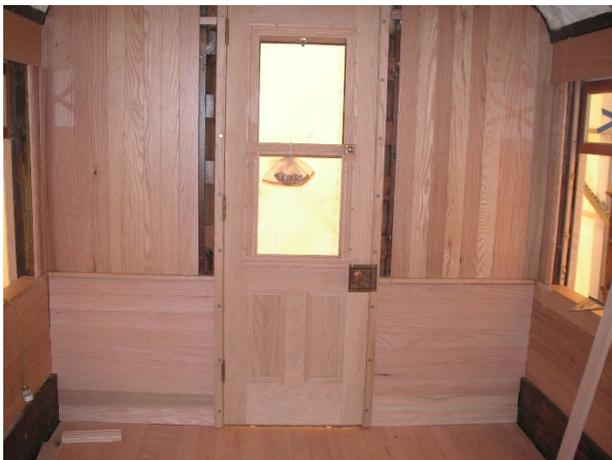
End walls in place, and door with original hardware
