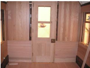
End walls in place, and door with original hardware
