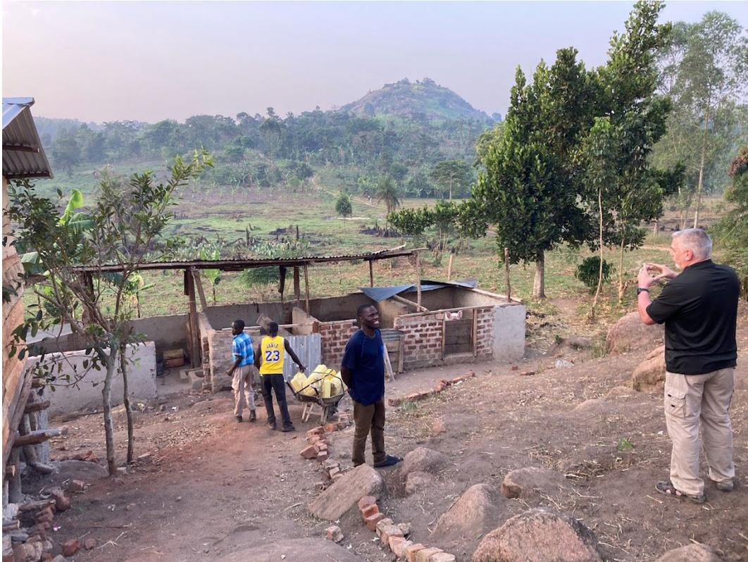
We will finish closing in this structure with concrete and boards and placing a chicken coop on top of the Piggery. Saves space and chicken manure helps with the pig food for the pigs.
