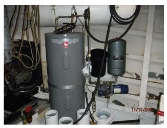
FRESHWATER ACCUMULATOR TANK Groco Accumulator Tank.
