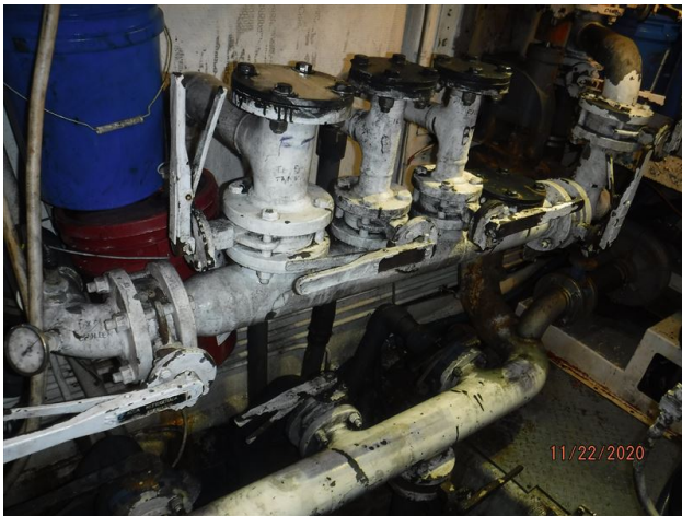
SEA CHEST MANIFOLD standard sea chest manifold design
