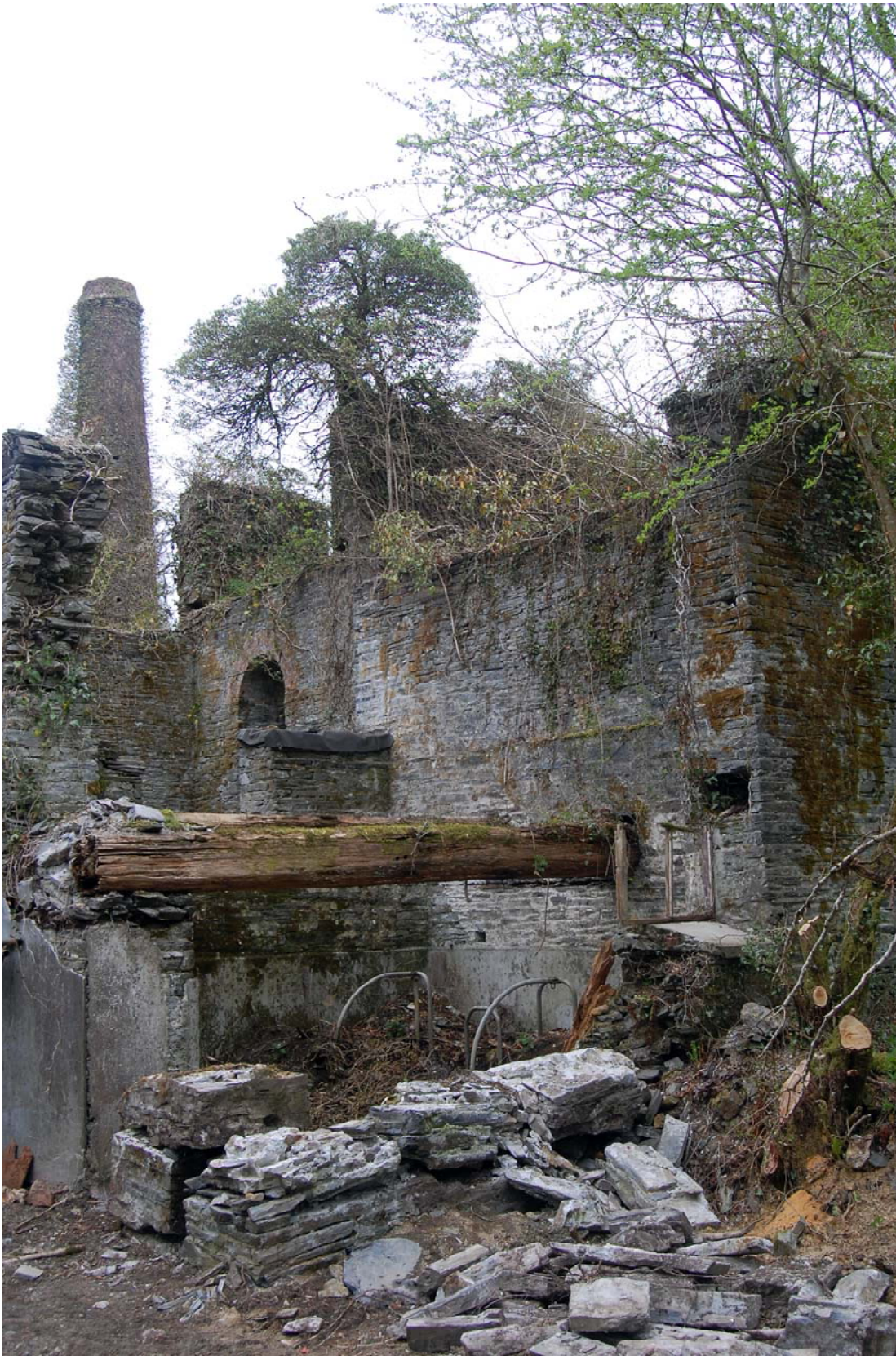
Crusher House at North Herodsfoot mine. April 2011. Roy Starkey photo.
