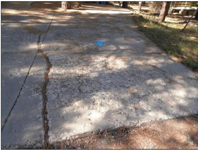
B. Item 1(Picture) Driveway salt damage
