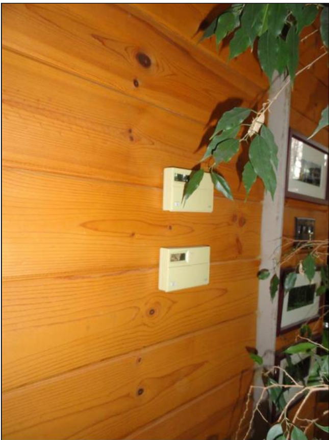
A. Item 2(Picture) Sunroom has 2 heating zones, floor and box radiators.
