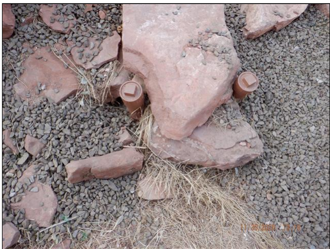
P. Item 2(Picture) two sewer clean outs next to the "sump pump"
