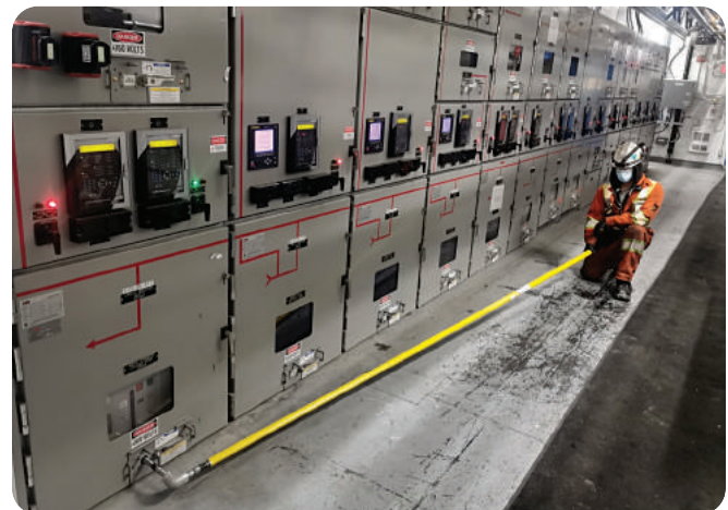
Xtend-a-Rack, extendable manual racking tool for power circuit breakers – This new product recently released by Amidyne Solutions moves the Qualified Electrical Worker up to 208 inches or approximately 17 feet away from the front of a power circuit breaker when it is racked in or out, eliminating exposure to arc flash or reducing the ATPV of ac flash PPE required.
