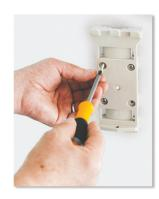
Secure the mounting bracket to the bulkhead.
