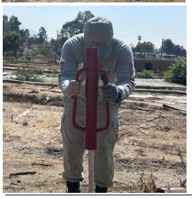
T Post Driver is used to start setting posts. Do not hit the wood posts too hard as they may split
