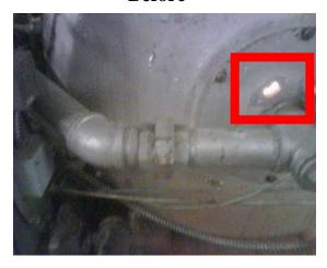
Before installing the PC Fuel Optimizer, the flame in the boiler combustion chamber view port is not as bright meaning fuel combustion is not optimal.
