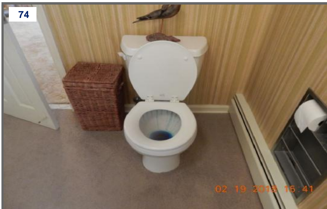
Master Bathroom is not functional. (2)
