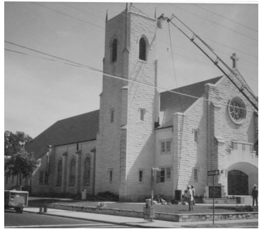
Sandblasting Cristo Rey Catholic Church, 1984.
