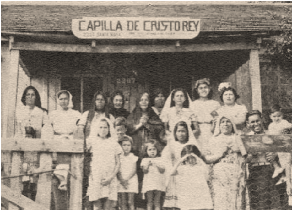
The Capilla de Cristo Rey at 2207 Santa Rosa Street.
