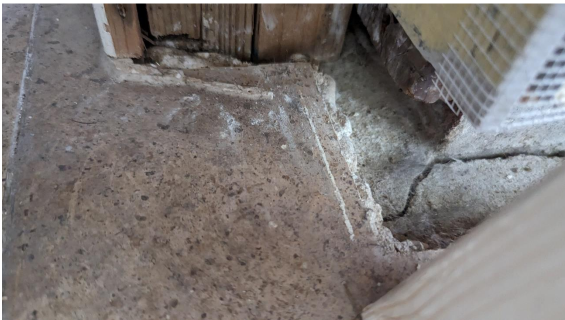
The foundation slab, where visible, is severely cracked at wall-floor joint.
