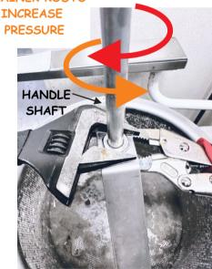
For proper button trap strainer seating adjust the length of the handle shaft. Using a channel lock or needle nose pliers to hold the lower locking nut and loosen the upper locking nut. Rotate the handle shaft while holding the upper locking nut to adjust the length of the handle shaft. When the correct handle shaft is adjusted properly, hold the upper locking nut and tighten the lower locking nut.
