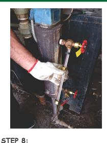
Insert the sight glass assembly into the upper fixture then slide it down into the lower fixture until it bottoms or is centered
