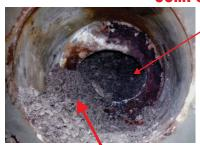
LOAD OF SCALE AT THE OPEN HAND HOLE ON A TURFUESS ROULER
