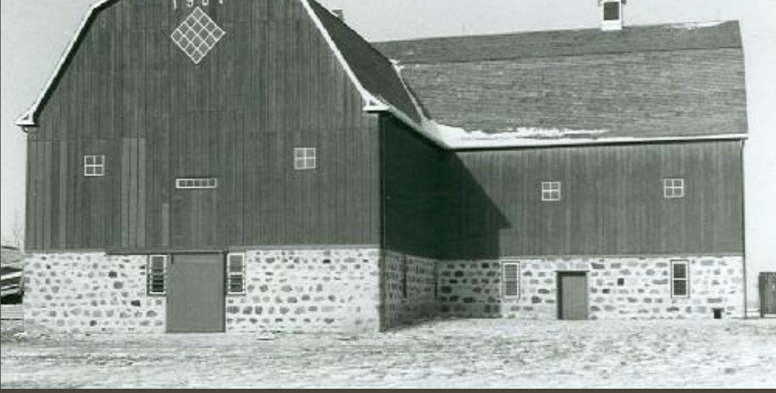
General view of the Barn, showing the L-shaped gambrel-roofed structure built of stone and timber, 1988. Agence Parcs Canada, Homestead Motherwell/ Parks Canada Agency, Motherwell Homestead, 1988.
